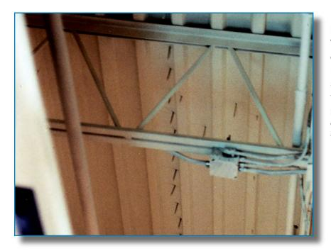
Figure 3-60: View of the underside of a steel deck showing the mechanically attached single-ply membrane fastener rows running parallel to, instead of across, the top flange of the deck.
