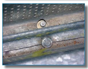
Figure 3-24: Looking down at a sidelap of a deck attached with powder-driven pins. The washer at the top pin blew through the deck.
