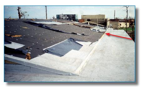
Figure 3-89: Mechanically attached single-ply membrane progressively tore after being cut by windborne debris. Hurricane Andrew (Florida, 1992)
