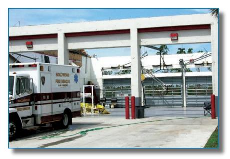
Figure 3-30: The roof structure over the apparatus bay blew off following the failure of sectional doors. Hurricane Charley (Florida, 2004)
