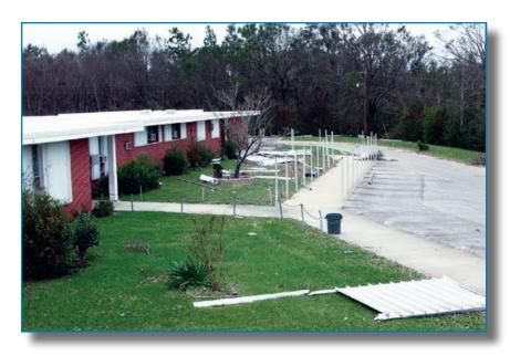
Figure 3-28: The destroyed walkway canopy in front of a school became wind-borne debris. Hurricane Ivan (Florida, 2004)
