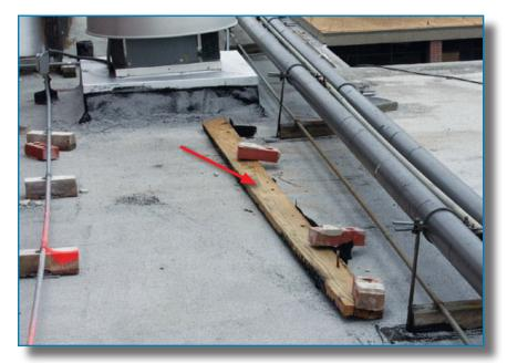
Figure 3-116: The edge nailer on top of an old brick wall at a hospital blew off because it was inadequately attached. Hurricane Ivan (Florida, 2004)
