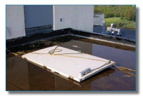
Figure 3-29: Door on a hospital penthouse blown off its hinges during Hurricane Katrina (Mississippi, 2005)
