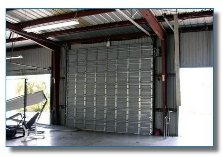
Figure 3-109: The new door in the center performed very well, but the older doors on either side of it were blown away. Hurricane Charley (Florida, 2004)
