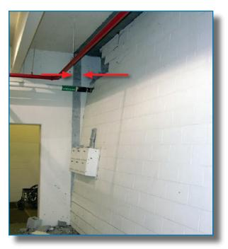
Figure 3-44: The red arrows show the original location of a CMU wall that nearly collapsed following a rolling door failure. Hurricane Charley (Florida, 2004)
