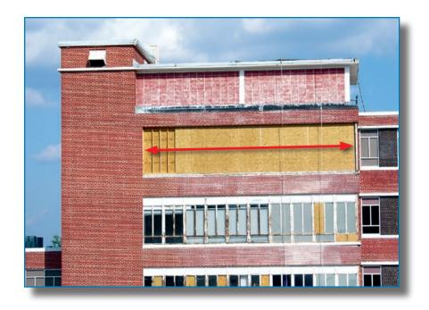
It is recommended that all non-impact-resistant, exterior glazing located in hurricane-prone regions (with a basic wind speed of 100 mph or greater) be replaced with impact-resistant glazing or be protected with shutters, as discussed in Section 3.4.3.2.
