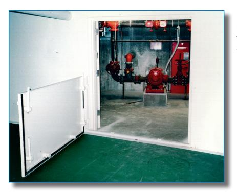
Figure 2-31: Equipment room with watertight door
