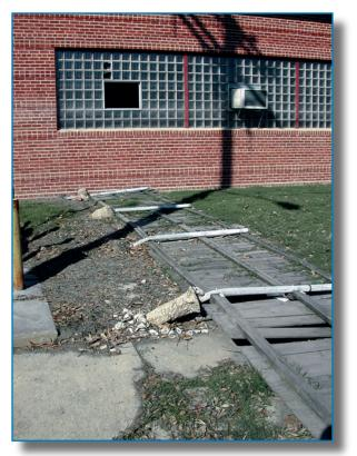
Figure 2-12: Katrina's storm surge flooding knocked down this fence adjacent to a fire station (2005).
