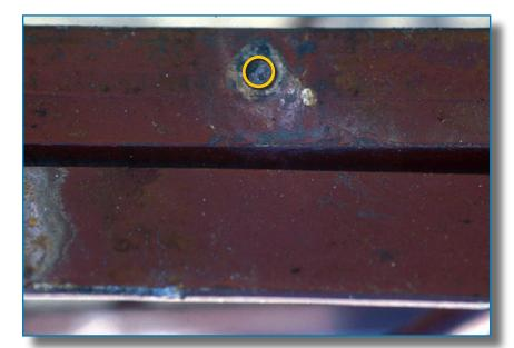
Figure 3-23: View looking down at the top of a steel joist after the metal decking blew away. Only a small portion of the deck was well fused to the joist (circled area). Tornado (Oklahoma, 1999)
