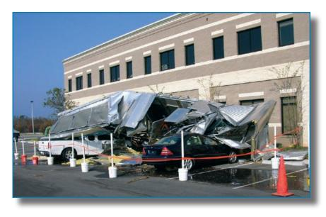
Figure 3-69: Although this 18,000pound HVAC unit was attached to its curb with 16 straps, it blew off during Hurricane Ivan. (Florida, 2004)
