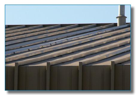
Figure 4-43: Lifted batten covers on Third District Fire Station metal roof
