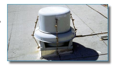
**Ductwork:** To avoid wind and wind-borne debris damage to rooftop ductwork, it is recommended that ductwork not be installed on the roof (see Figure 3-72). If ductwork is installed on the roof, it is recommended that the ducts' gauge and the method of attachment be able to resist the design wind loads.
