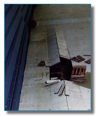
Figure 2-17: This parquet wood gymnasium floor was damaged by dimensional changes due to saturation. Hurricane Katrina (2005)
