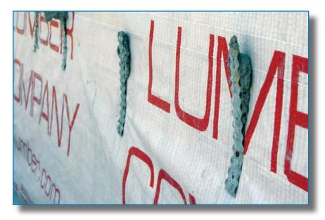
Figure 3-47: These four ties were never embedded into the mortar joint.
