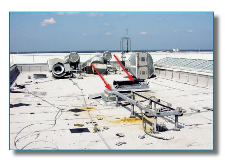
Figure 3-20: Temporary coverings placed over two large openings in the roof that were left after the ductwork blew away. Hurricane Katrina (Mississippi, 2005)
