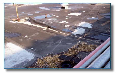
Figure 4-7: Roof membrane starting to peel off at Hancock Medical Center.
