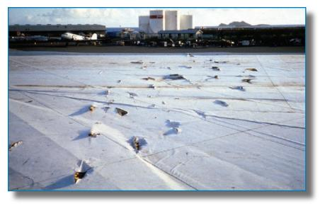
Figure 3-90: Fully adhered single-ply roof membrane struck by a large number of missiles. Hurricane Marilyn (U.S. Virgin Islands, 1995)
