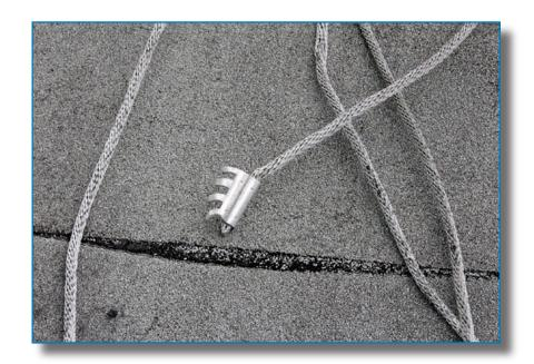
Figure 3-101: Bolted splice connectors are recommended to prevent free ends of connectors from being whipped around by wind. Hurricane Katrina (Mississippi, 2005)
