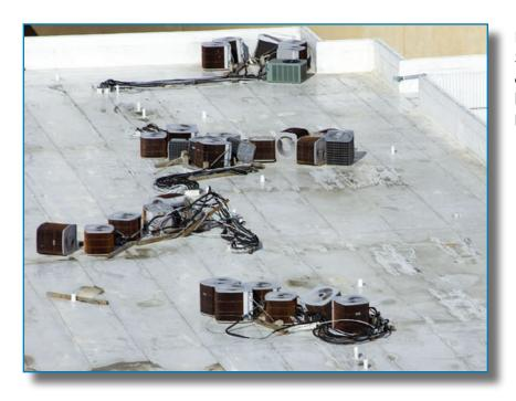
Figure 3-73: Sleeper-mounted condensers displaced by high winds. Hurricane Katrina (Mississippi, 2005)
