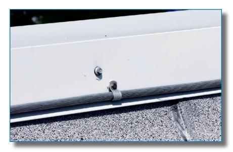
Figure 3-97: This conductor was attached to the coping with a looped connector. Hurricane Katrina (Mississippi, 2005)
