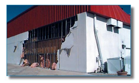
Figure 3-55: EIFS blown off a cast-inplace concrete wall. Note the damaged rooftop ductwork. Hurricane Ivan (Florida, 2004)
