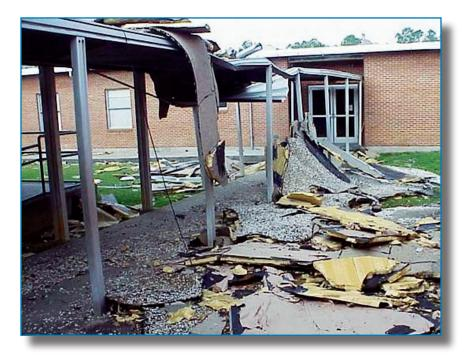
Figure 3-83: Open walkways do not provide protection from wind-borne debris. Hurricane Katrina (Mississippi, 2005)
