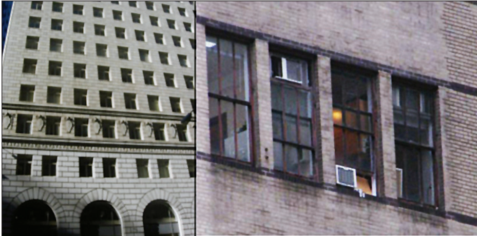
Figure 3-43: Punched windows (left), ribbon windows (right)
