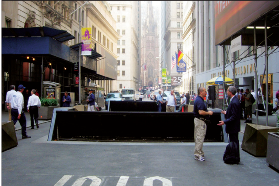
Figure 2-25: Sally port installation with two active barriers
