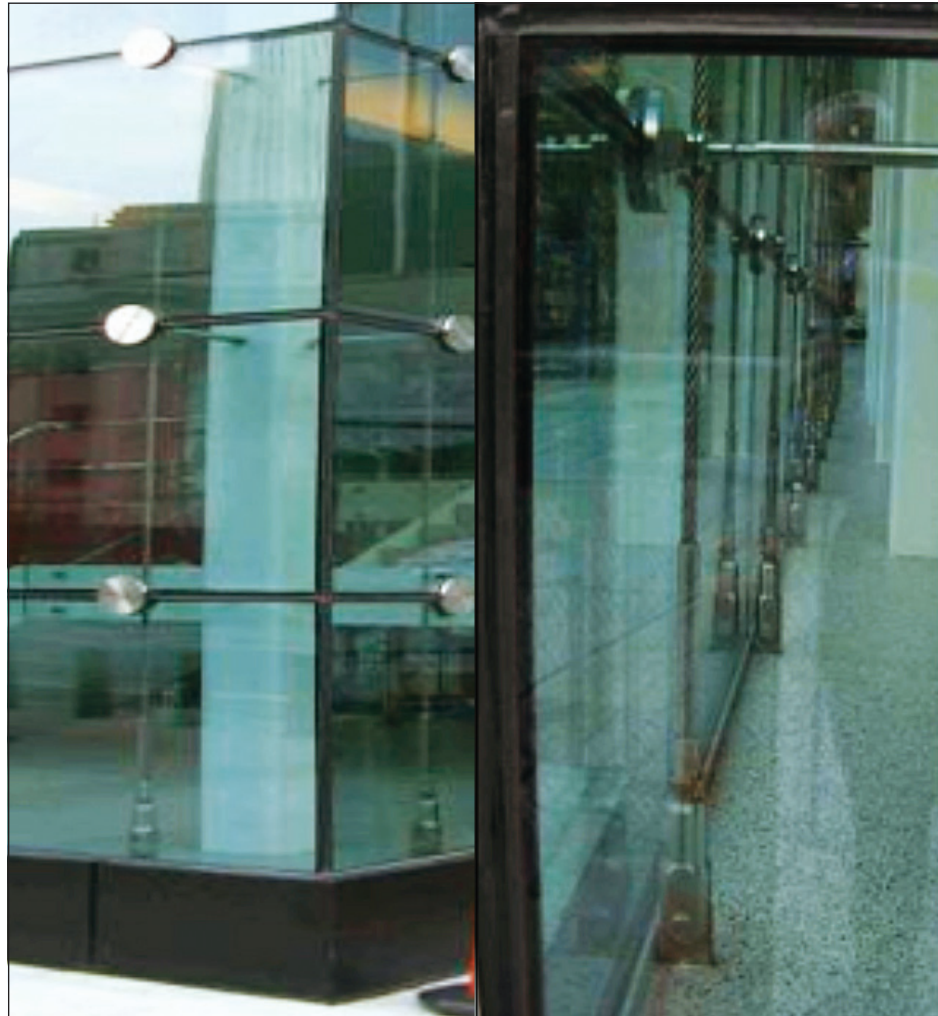
Figure 3-53: Example of cable catch system
