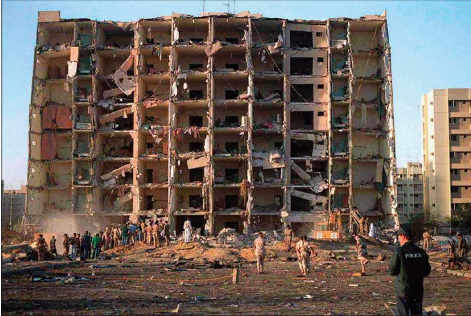
Figure 3-36: Khobar Towers, Dhahran, Saudi Arabia, 1996
