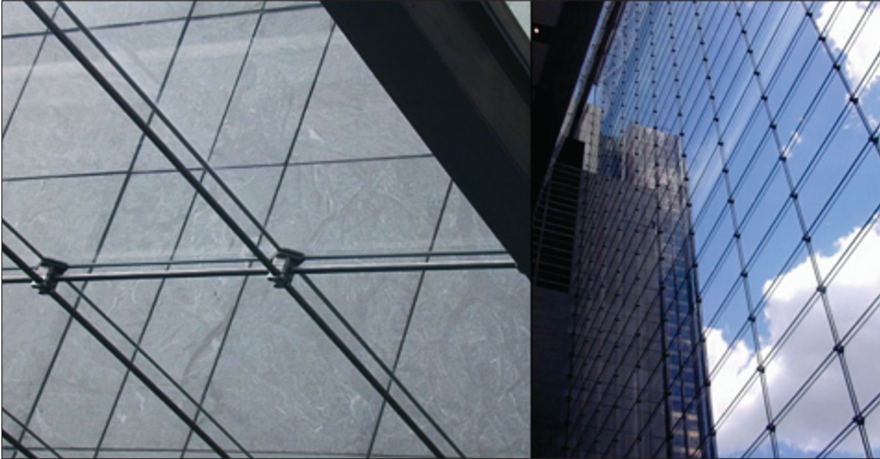
Figure 3-50: Point- and cable-supported curtain wall
