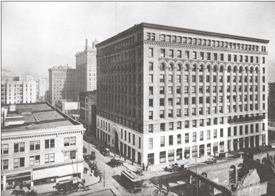
Figure 3-37: Mills Building, San Francisco, 1891, steel frame with URM infill
