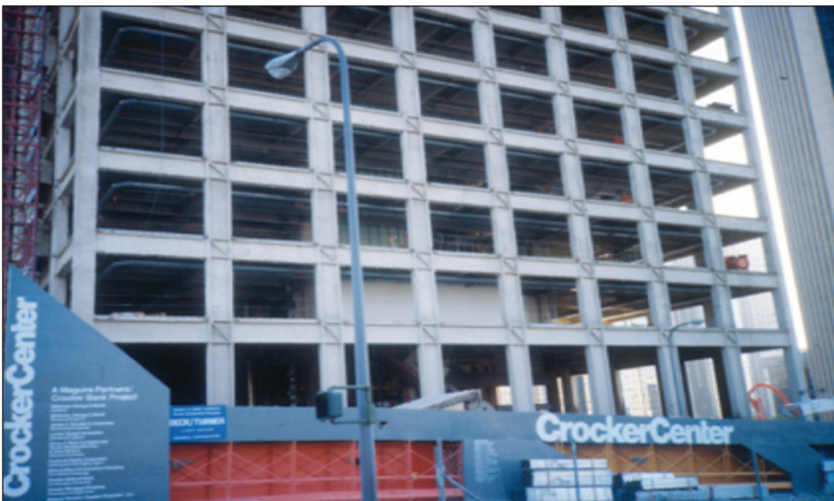
Figure 3-33: Moment-resistant steel frame structure
