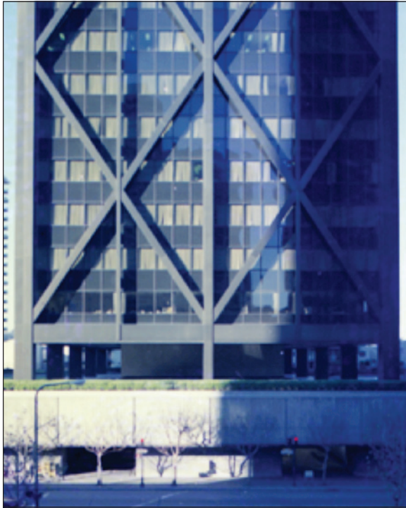
Figure 3-34: Exposed steel braced frame
