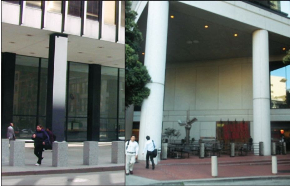
Figure 3-42: Exposed perimeter column (left), exposed columns supporting end of building (right)
